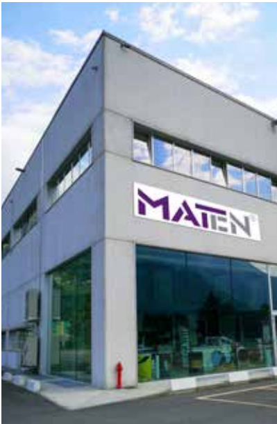
The new operational HQ Mat.en in Artogne (BS)
